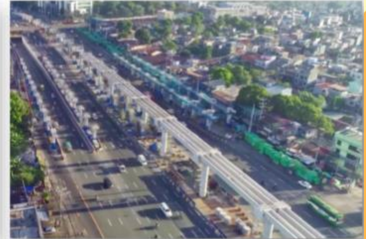
METRO MANILA RAIL TRANSIT SYSTEM LINE 7 (MRT-7)
