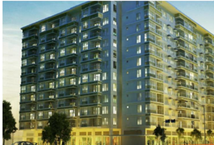
Veranda by Alveo
