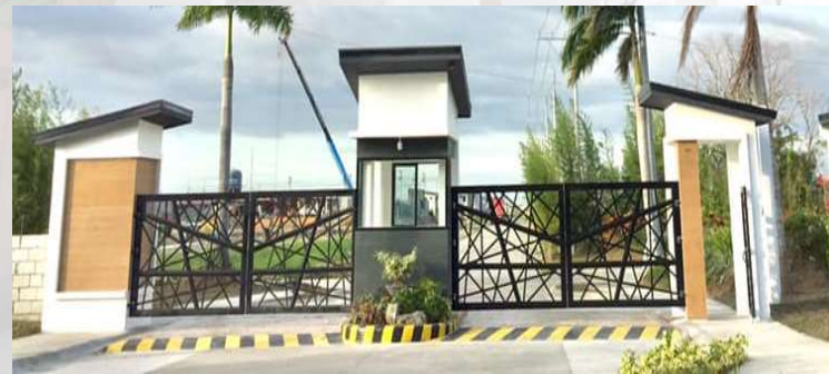
Main Gate with CCTV Camera & Guard House manned 24/7
