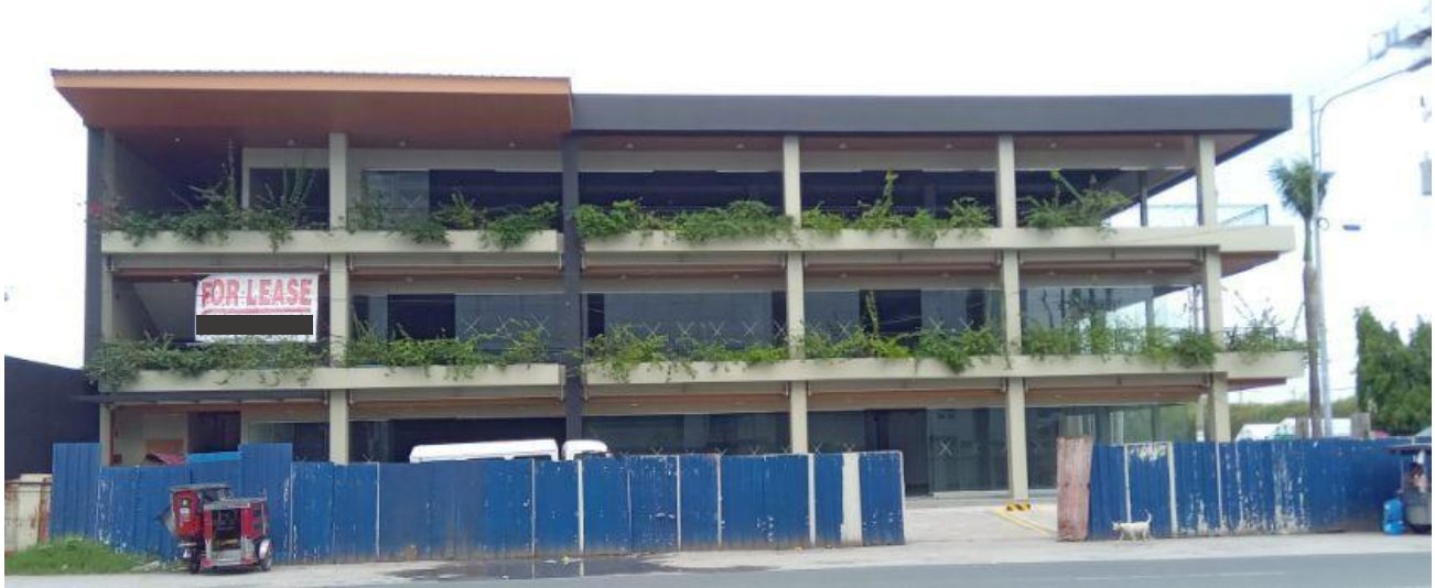
BUILDING CONSTRUCTION DONE AS OF AUGUST 2024
